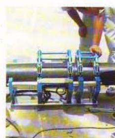
Leave the pipes to cool down for a period as calculated. Maintain pipe ends' pressure level during cooling period.
