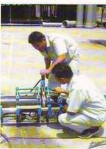
Press both pipe ends toward the Heater Plate when the plate's temperature is appropriate. Apply pressure as calculated to produce beads with the right size.
